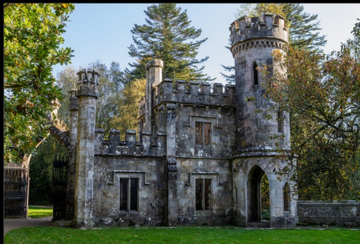
VO-M-Hannes Van Den Berg-36-G-Irish Tower At Ballysaggartmore
